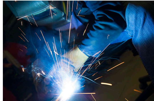
On-Site coded welders
